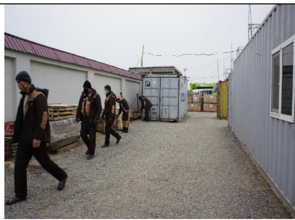
Figure 12. The construction camp is covered with crashed stone and the cleanliness of the territory is observed.
