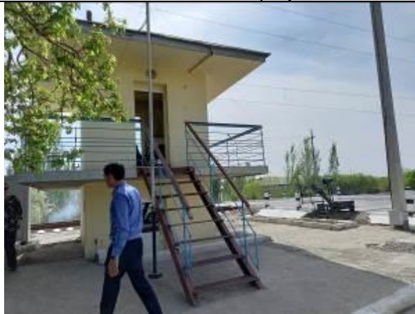
Figure 2. Protected level-crossing “52 nd km” (2022)
